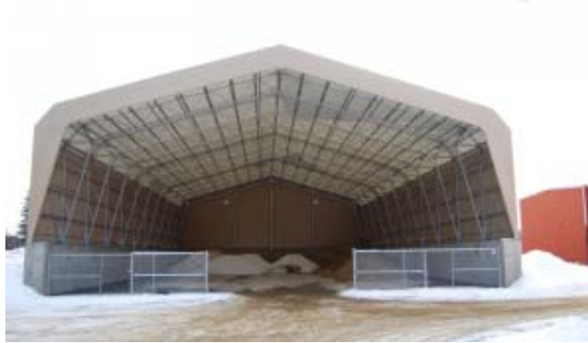
Figure 27. Town of Derry NH Salt Storage
